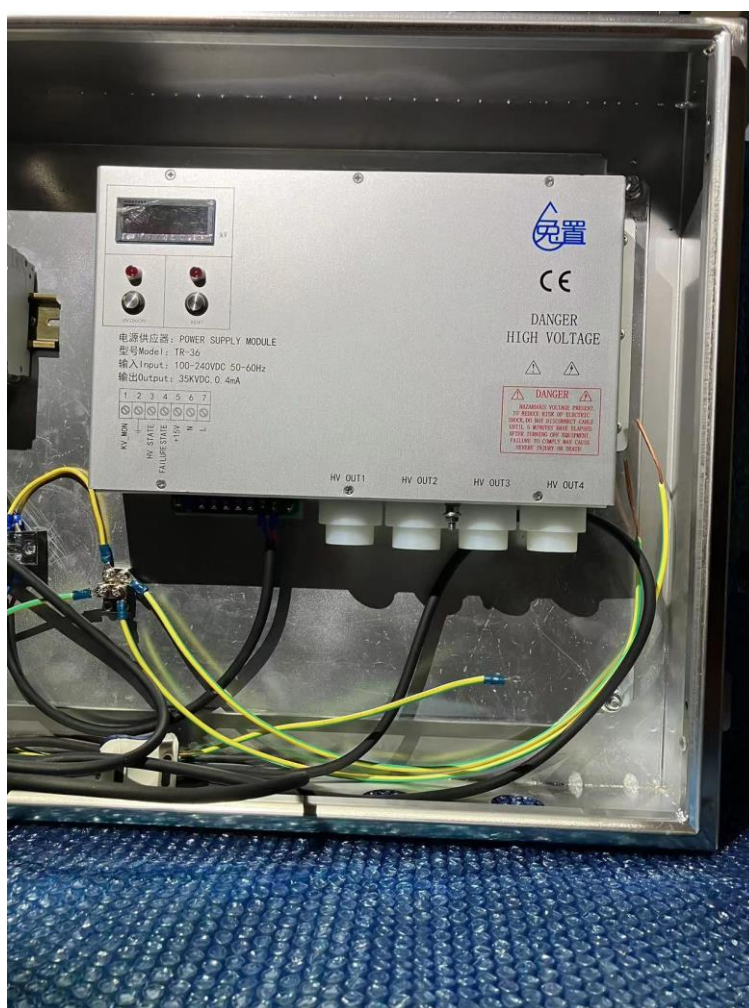
Figure6-1 Picture of distribution box without high voltage output connectors
